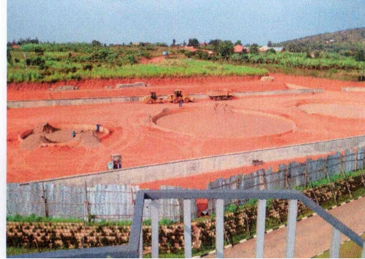
Bund wall and ring-beam foundation for a tank farm
