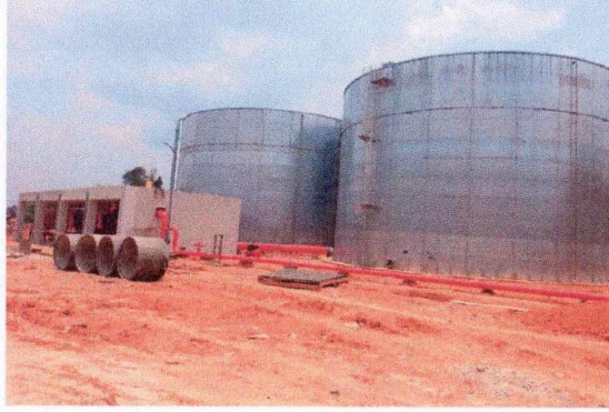
Completed firewater tank foundations
