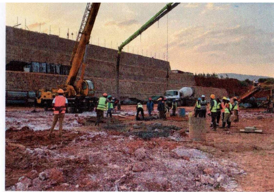
6 m retaining wall under construction — depot platform
