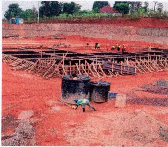
Construction of bottling hall for LPG cylinders
