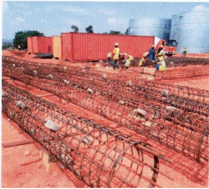
Pile cage reinforcement for tank foundation
